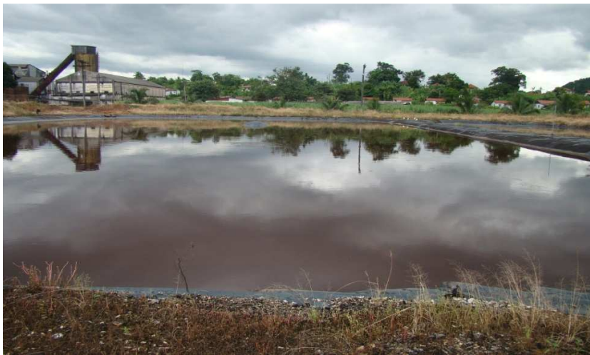
Dunder Ponds Exceed Design Holding Capacity and Spill To the Environment Photo Taken July 2010
