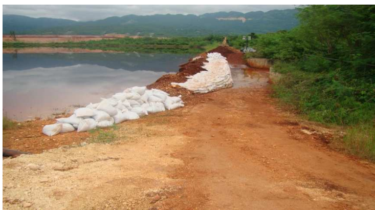
Caustic Effluent in the Holding Pond at Ewarton Works, Charlemont, St Catherine Exceeds its holding capacity and overflows via the spillway. Sand bags used to obstruct flow through the spillway. Photo taken October 2010
