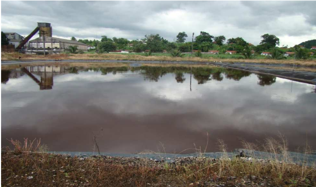
Dunder Ponds Exceed Design Holding Capacity and Spill To the Environment Photo Taken July 2010
