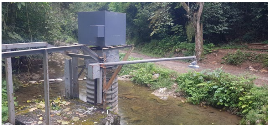
River gauging station on the Rio Doro at Williamsfield, St. Catherine upgraded with radar sensor and eTracker
