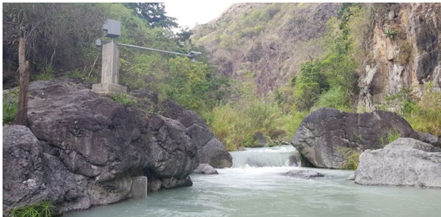
Figure 6: New Station constructed on the Yallahs River at Ramble, St. Thomas
