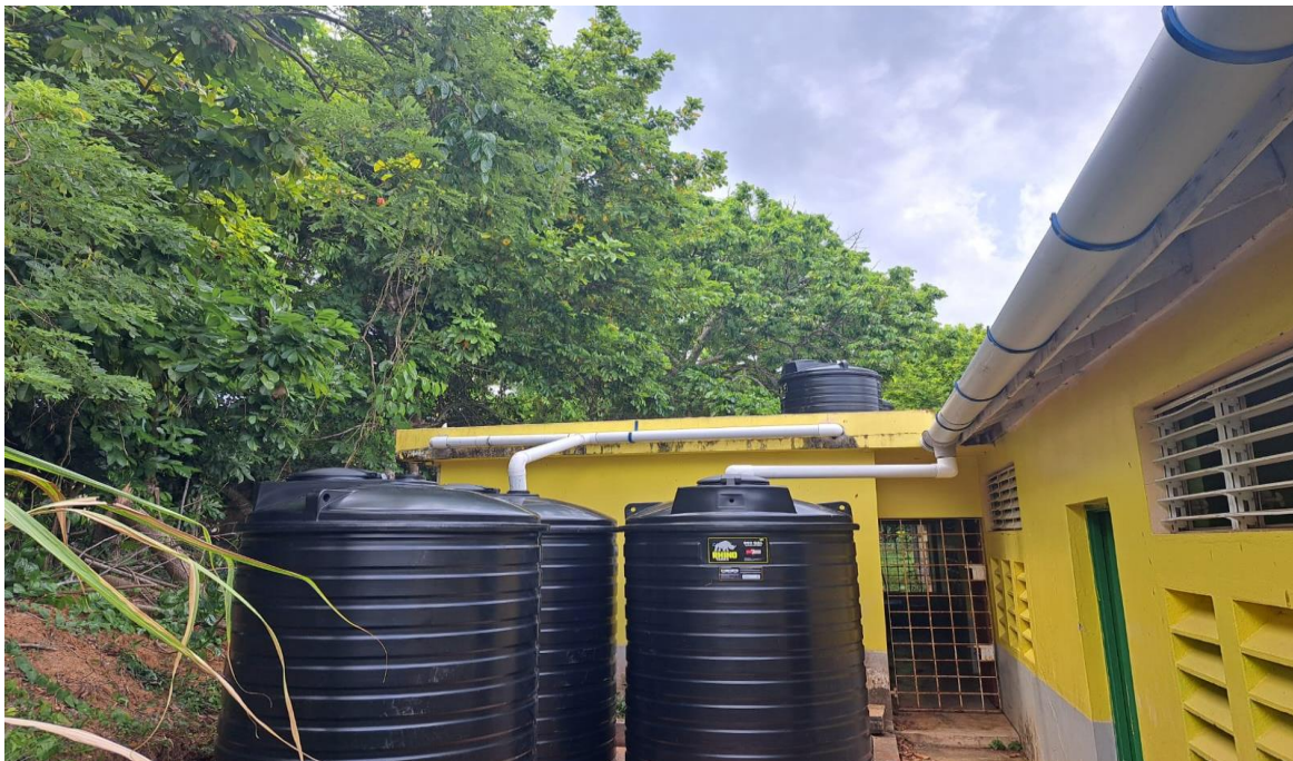
Picture 4: Wood Hall Basic School Rainwater Harvesting System - Clarendon (Courtesy of Rural Water Supply Limited)
