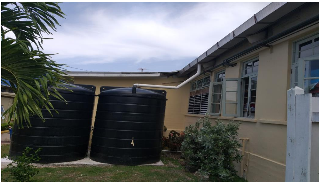
Picture 1 & 2: St. Anns Bay Hospital Rainwater Harvesting System - St. Ann (Courtesy of Rural Water Supply Limited)
